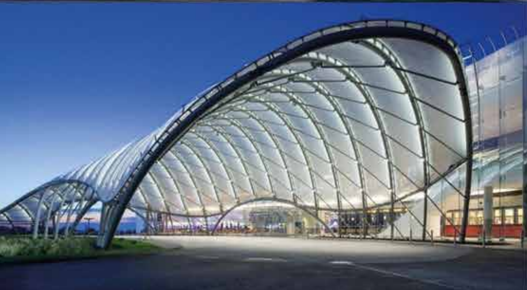
Maison a Lyon Vaise 1987, Jourda&Perraudin, Francia (Photo Jourda&Perraudin Archive). Law tennis Association Roehampton Hopkins Architects 2008 (Photo Hopkins Architects Archive). Empire City Casino Shelter ETFE Yonkers New York, FTL Nic Goldsmith (FTL Archive).
